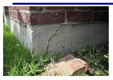
□ Note structural issues of the foundation such as sinking, water marks, cracking or flaking
