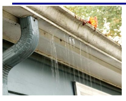
☐ Inspect gutters and downspouts for proper drainage, gutter slopes toward downspouts and is adequately secured
